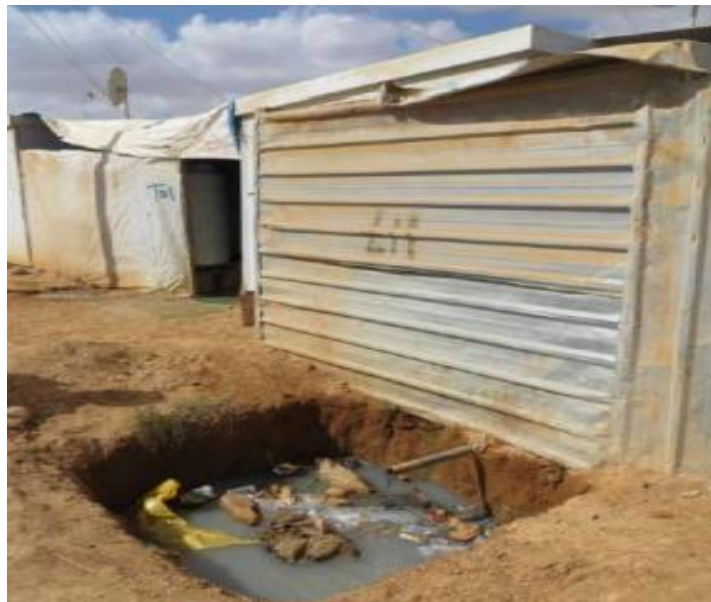
Figure 6. Wastewater storage pit (ACTED, JEN, OXFAM, UNICEF, et al., 2014)
