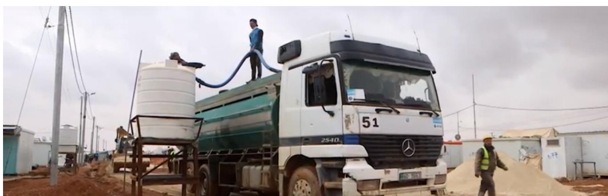
Figure 5. Water truck filling water storage tank. Picture is a screenshot from a KFW movie (2018)
