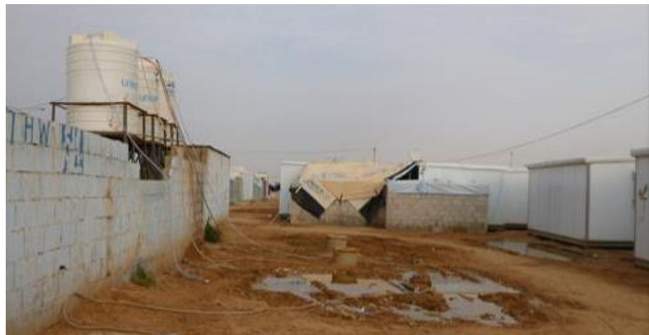
Figure 15. Private hoses connected to public water storage facilities. Picture derived from ACTED et al. (2014)
