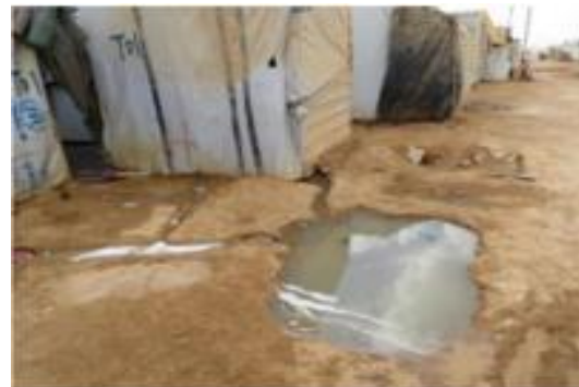
Figure 16. Ditches connected to a wastewater pit. Picture from (REACH; UNICEF, 2014a)
