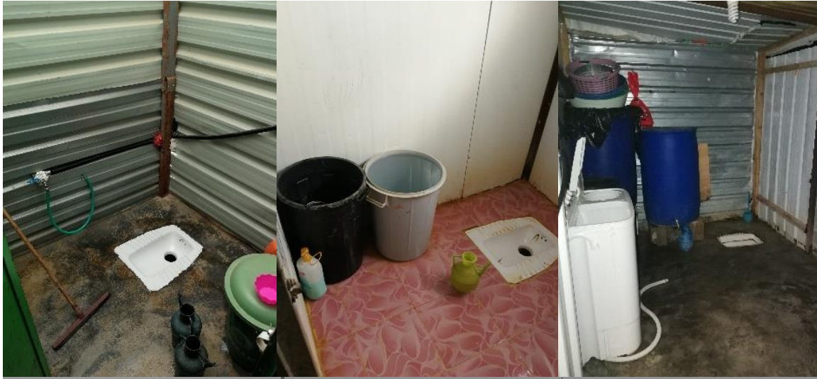
Figure 18. Current private toilet facilities. All pictures made by author
